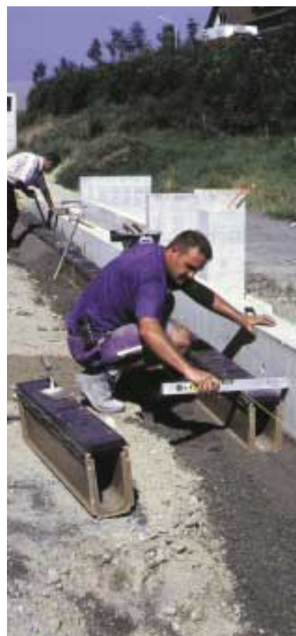
Channel installation
